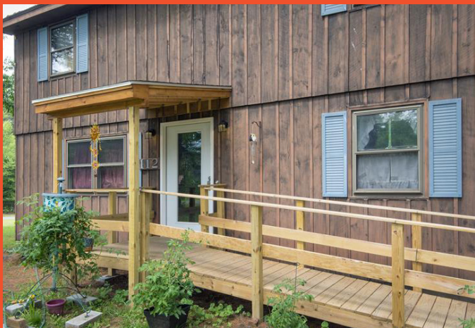
A ramp funded by the HMLP program in Southampton. Photo courtesy of CEDAC.
